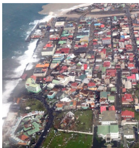
Hurricane Maria in Dominica (2017)
