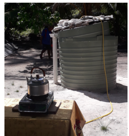
A bio-digester produces methane from piggery waste in Funafuti, Tuvalu (SPC, 2022)
